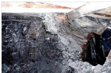
Fig. 6. Condition of rock mass around the gateroad at the "Stepova" mine – phenomenon of rib bending
