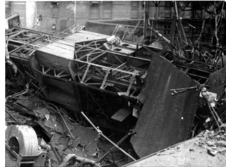
**Fig. 2.** View of the collapsed headframe in the "Bolesław" shaft in the "Bobrek" colliery (Lecomte et al., 2012)
