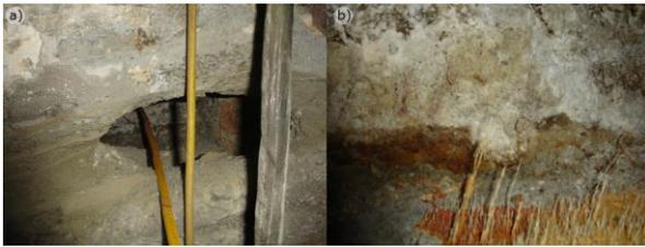
Fig. 5. The void behind the shaft lining: a – the opening in the lining with dimension of approximately 0.05 × 0.10 m, b – the roof of the void with visible corrosion products
