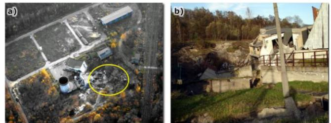
**Fig. 3.** The catastrophe of shaft "V" in the Knurów-Szczygłowice coal mine: a – general view of the scene of the catastrophe from the north (the crater area is marked yellow), b – damaged nearby buildings (Prusek, Bock, Uszko, & Dziura, 2013)
